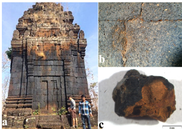
Figure 1. a) Neang Khmoa Temple (South exposition); b) detail of the stone surface; c) stereomicroscope sample observation
